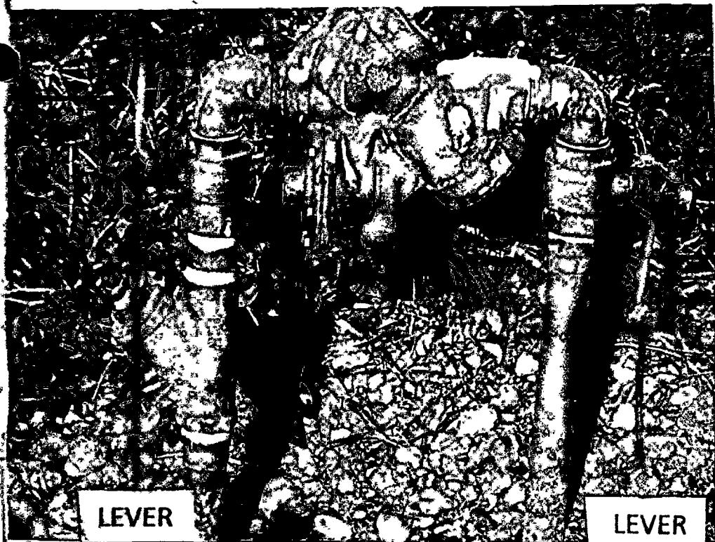
TURN ANY ONE OF THE TWO LEVERS INTO THE HORIZONTAL POSITION TO SHUT OFF WATER
